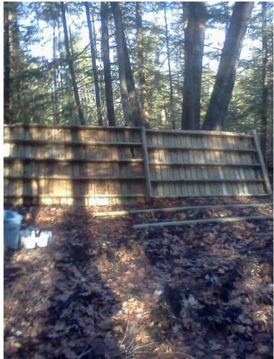
full length view of the bridge
